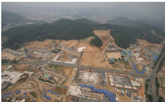
Figure 1. The complete view of excavation region within Eunpyeong Newtown.
