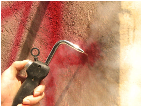
Figure 9. Application of low pressure steam cleaning for the Samjeondobi Monument.
