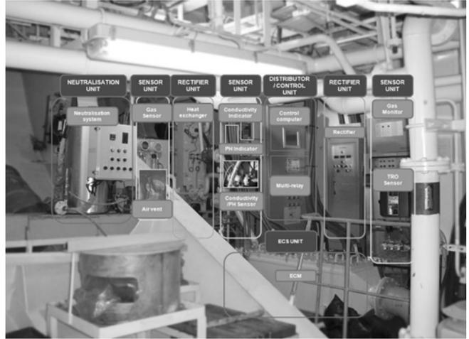
Fig. 5. Electro-Clean™, System of M/V Yokohama.
