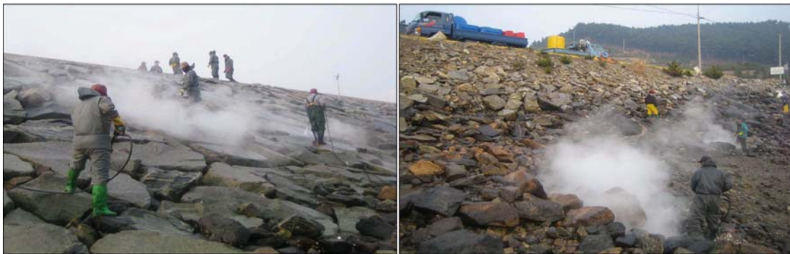
Fig. 9. Images of application of high-pressure warm water at Iwon tide embankment for oil recovery used at the oil-polluted Taean coastal area in January 6, 2008.
