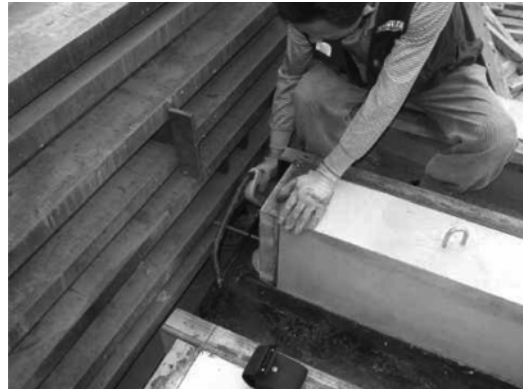
Fig. 9 Prestressing release
