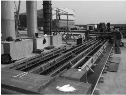
Fig. 5 Steel and CFRP tendon setting
