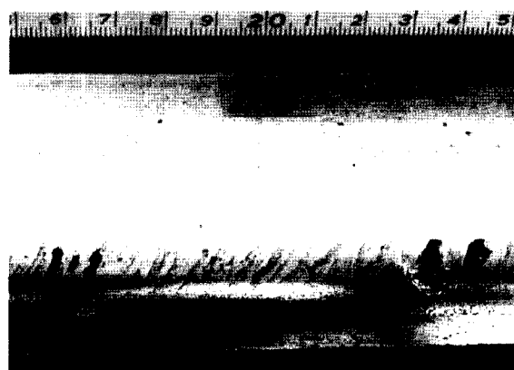
Fig. 1 Rail Head Checks on Outer Rail
