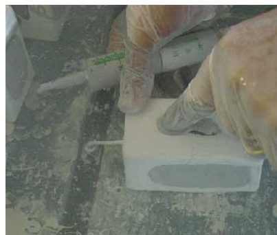
Fig. 2. Repair coat in water
