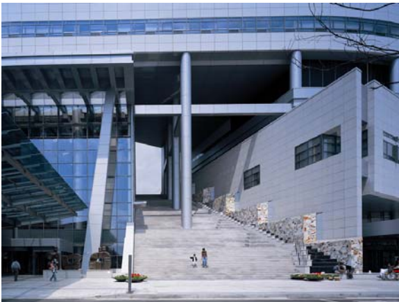
Figure 14. New Yonsei Severance Hospital - Grand Stairway
