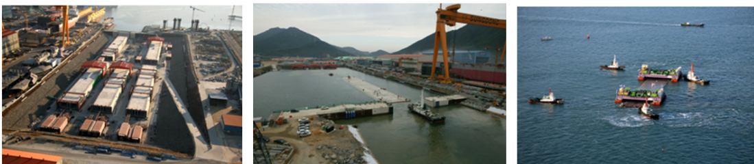
Fig. 7. The features of floating and transportation of caissons
