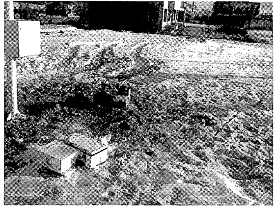
Fig. 3. Photograph of field installation.
