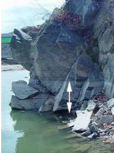
Fig. 10. Falling Down of Water Level after the Weir Removal (Left Hand Side of the Stream and just Upstream of the Weir)
