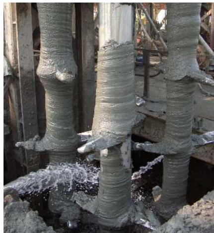
Fig. 2 Mixing equipment of D.C.M method
