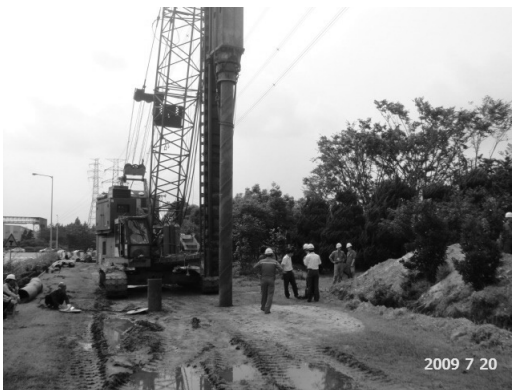
Fig. 1. View of pile driving.
