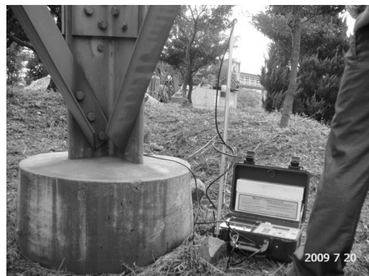
Fig. 2. View measuring of the Power line tower base.
