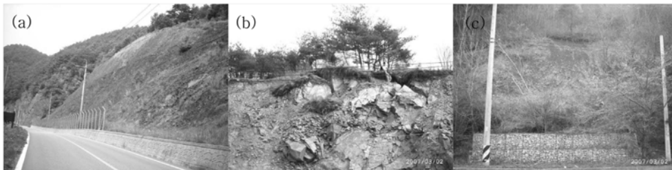
Fig. 1. Most representative pictures of the study area. (a) MW-1 site : non-failure slope, (b) CJ-2 : failure slope, (c) CJ-3 : circular failure.
