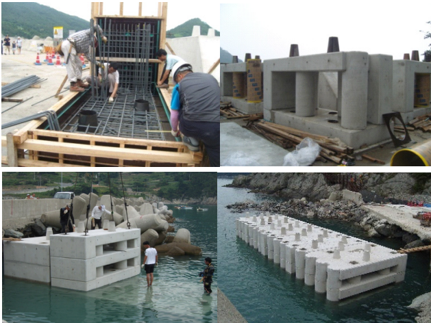
Fig. 12 Field construction and installation of units and structures
