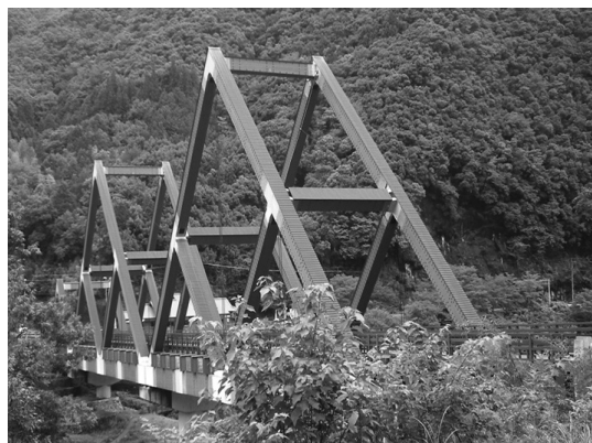
(b) Karikobou Bridge
