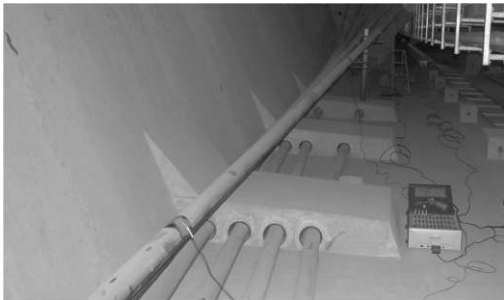
Photo 1 The picture of field test(Seohae Bridge)
