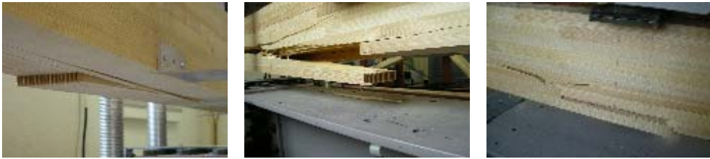
Fig. 15. Breaking shape of Composite material beam.
