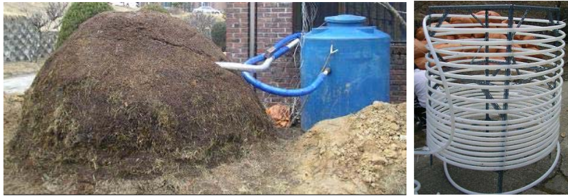
Fig. 1. Fermenting beds and pipe installation (helical type) for heat exchanger.
