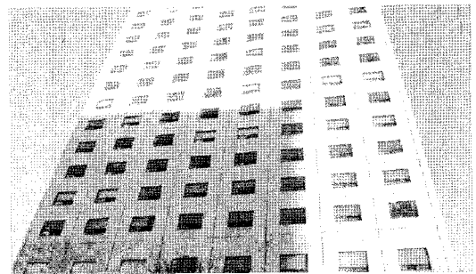
Figure 11. None exterior stairs of Hospital Bldg.
