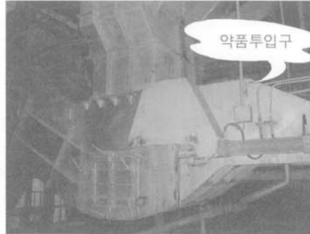
(Fig. 4) Chemicals injection system from Ash Extractor.(1 step)
