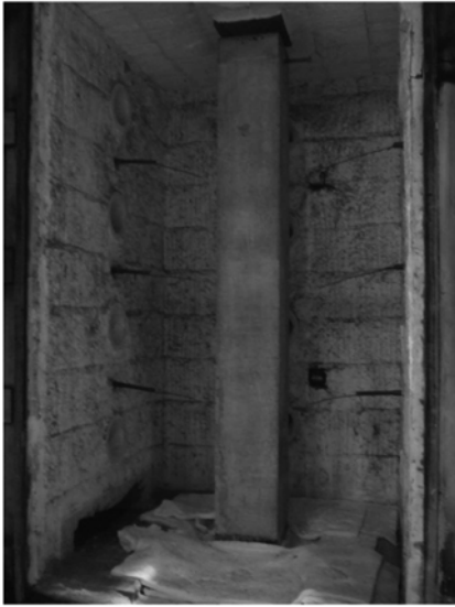
Fig. 7 Appearance of specimen after fire test
