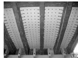
Lower surface of Concrete Road Slab
