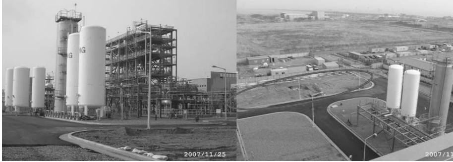
DME Demo Plant
