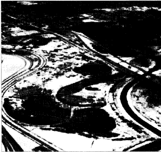
(a) Aerial View Pre Construction (O'Meara et al, 2002-2003)
