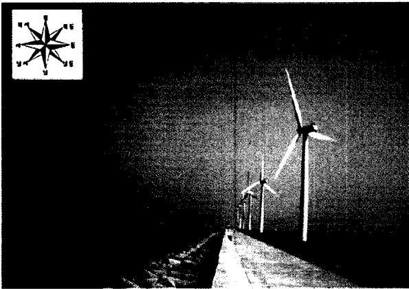
Photo 1. 850kW class wind generator at Bieungdo of Gunsan.
