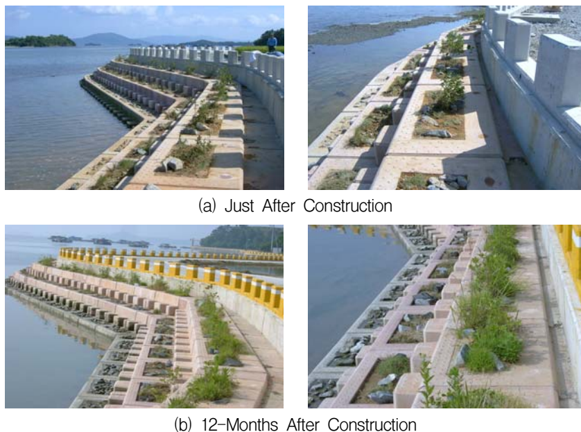
Fig. 6. Field Experiment for Vegetation Culture in Shore
