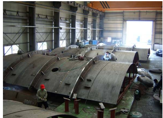
Figure 5. Manufacture of Vacuum vessel
