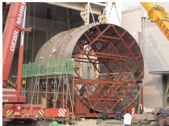
Figure 6. Assembly of Vacuum vessel
