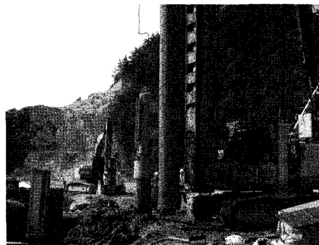
Fig. 1 PRD equipment and auger working stage
