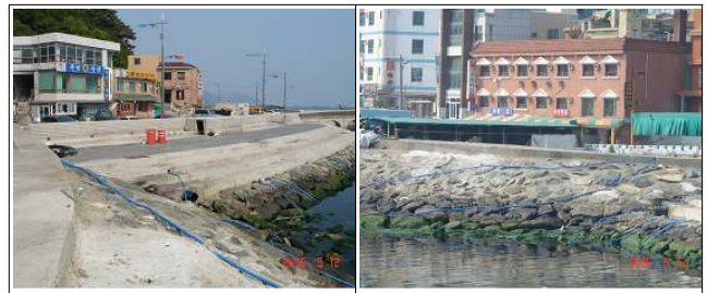
Photo 11. Songdo area with ocean water pumping system in Busan city.
