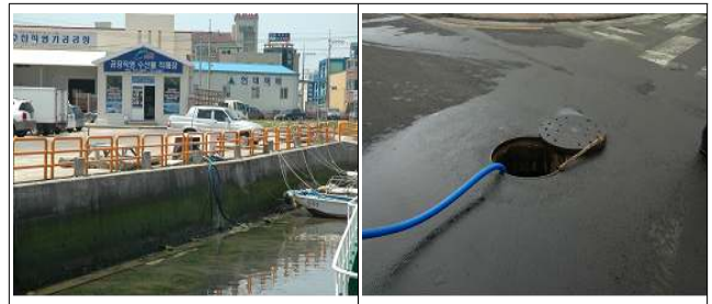
Photo 5. Doduhang area with ocean water pumping system in Jeju city.
