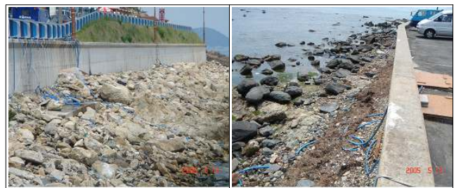
Photo 12. Cheongsapo area with ocean water pumping system in Busan city.
