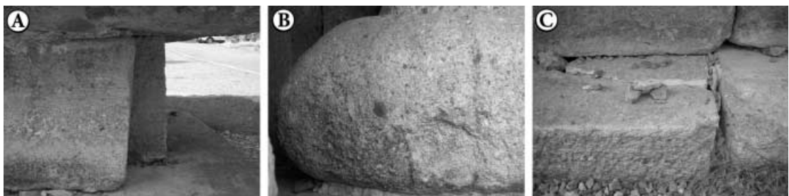
Figure 7. Representative physical weathering of host rocks for the store Budtlhas and Shire. (A) Northern under base rocks show partly fractured and exfoliated. (B) Rounded exfoliation developed on surface of the Buddha store. (C) Eastern flat stones show fractured and fragmentation.
