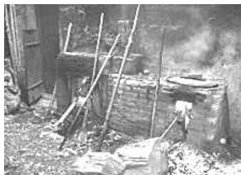
⑨ Heating up drying board
