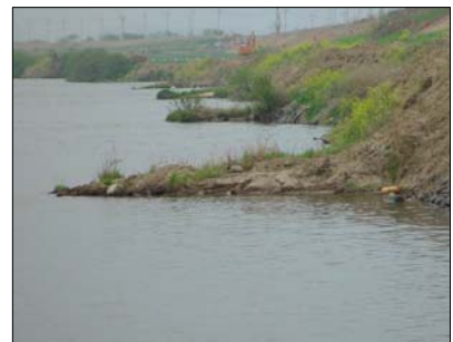
Fig. 3. Lmpermeable Groyne (NakDong river)
