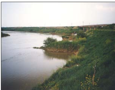
Fig. 1. Lmpermeable Groyne (YoungSan river)
