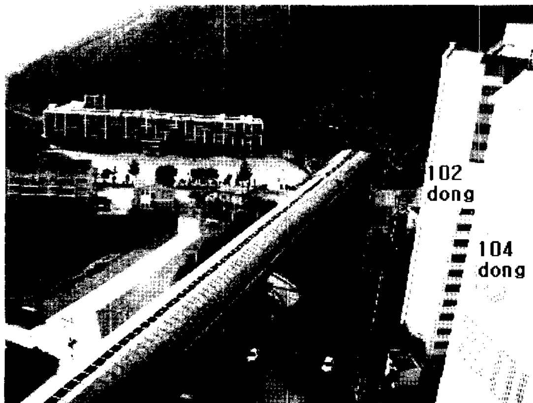
Photo. 1 The scene of sound absorption tunnel on the elevated railway
