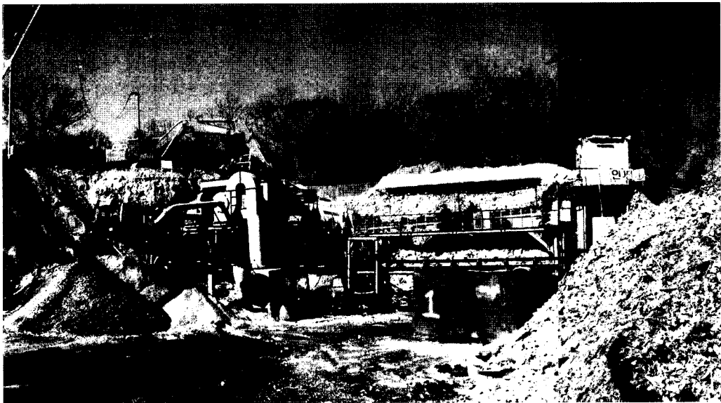
Fig. 9. Processing view of the mixed construction waste in S. Environmental Co.
