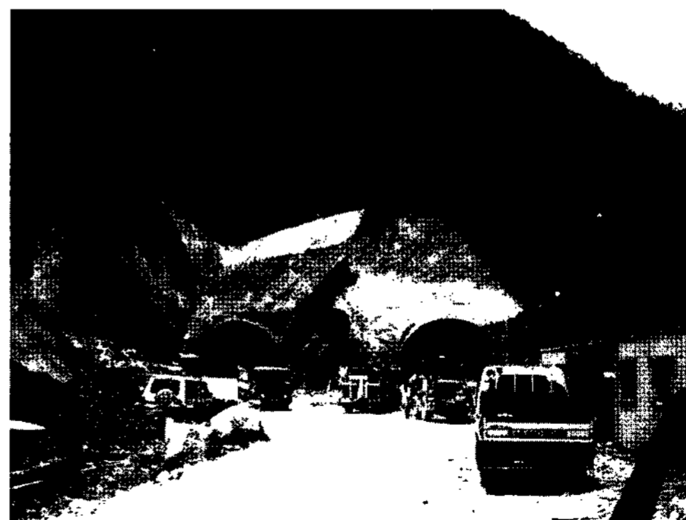
Fig. 6. View of the OO tunnel in Chubu-Myun.
