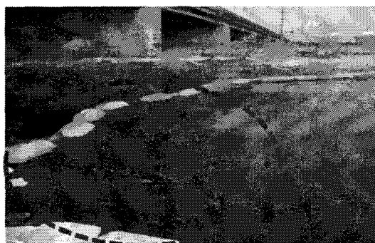
Fig. 6. Picture of oil girdle formed with installation of buoy.
