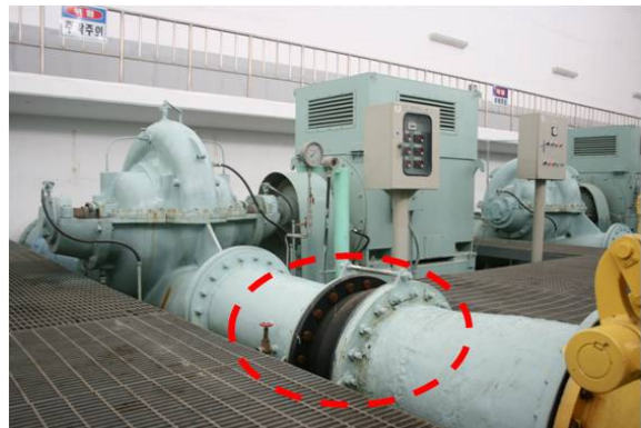
Fig. 3 Actually installed bellows location
