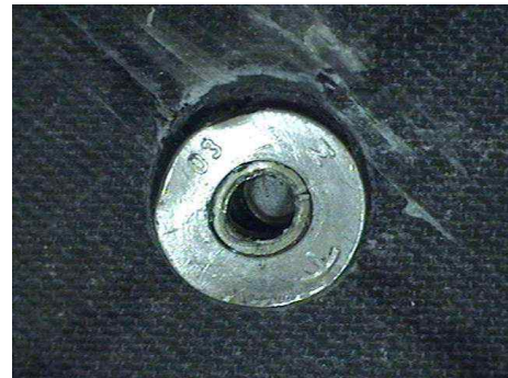
Fig. 14. Rivet (head) failure
