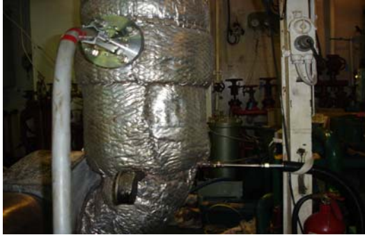
(b) Probe position for M/E NO x and smoke measurement
