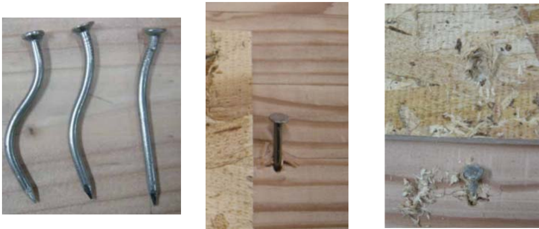
Fig. 6. Failures of nails and tested specimens.
