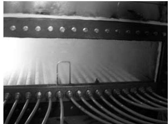
Fig. 3. Array of alumina ceramic membrane diffusers in air flotation tank.
