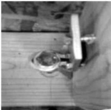
(a) Failure of applied lag screw
