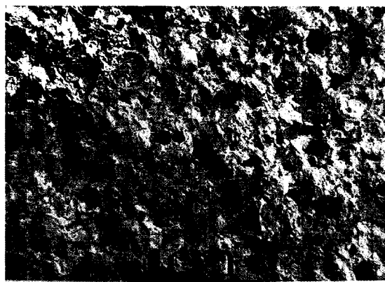
Fig. 2. Stone surface of the West Stone Pagoda of Gameunsa Temple Site. A, B, C, and D indicate mineral fragments of quartz, feldspar (altered), hornblende (removed), and biotite (hexagonal shape), respectively.
