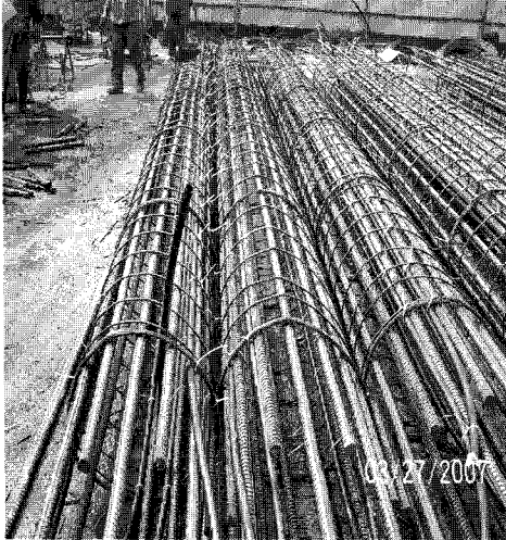
Fig. 2. View of pile foundations before casted and buried.
