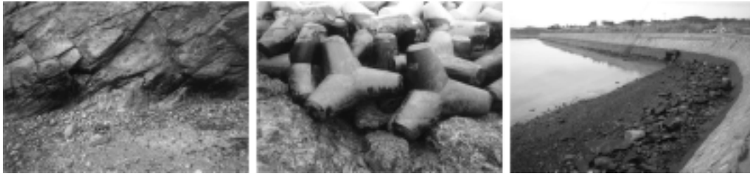
Fig. 14. Photos of oil adhesion on rock(a), tetrapod(b) and artificial revetment(c) at Taejan in December 12.
