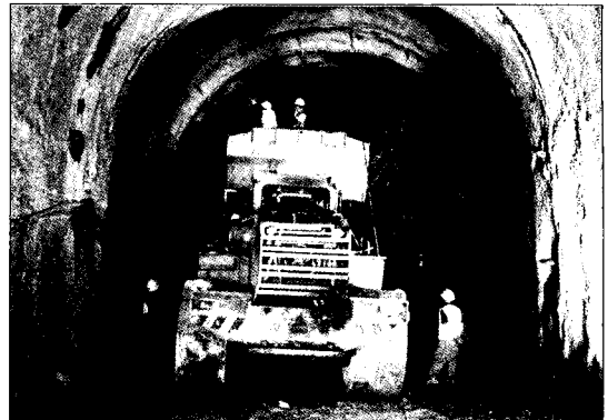
Fig. 19. View of installing the rockbolt
