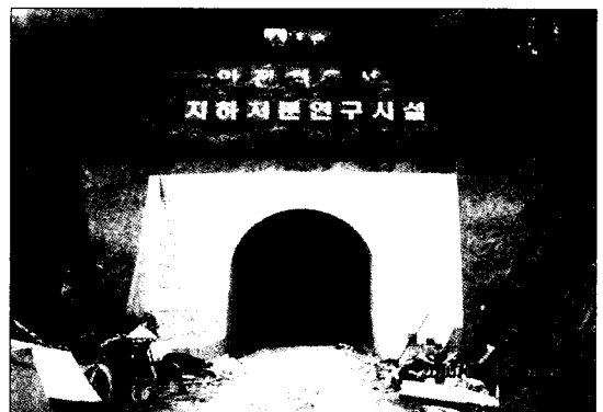
Fig. 21. View of the construction of the portal
