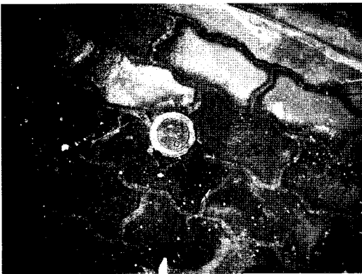
Fig. 6. Buried gas pipe line in an acid drainage generating earth.
