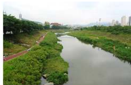
(5) Improving the straight channel (considers the mobility of riverbed materials)
