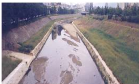
(5) Improving the straight channel (considers the mobility of riverbed materials)
