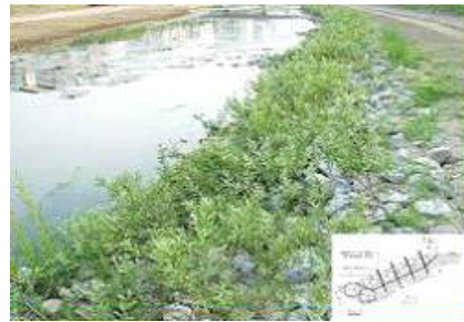
(2) Forming gently-declined revetment
