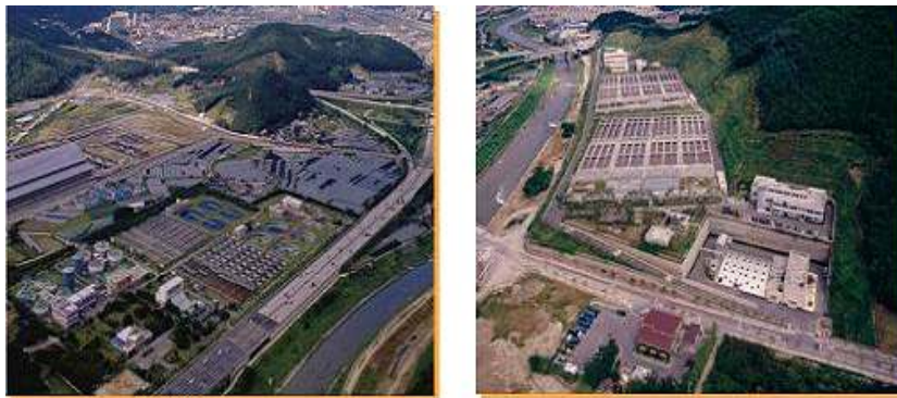
Figure 4. Sewage Treatment Plants (Left : Bakdal Plants established in 1995/Right : Seoksu Plants established in 2002).
