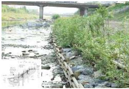
(1) Forming revetments using natural materials
