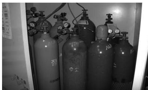
Fig. 3. Mixed storage of compressed gas cylinders in the gas cabinet.
